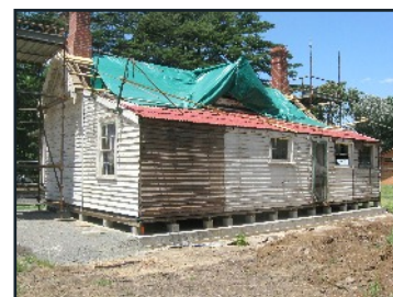
Developments at the Gatekeepers Cottage: Now re-stumped on the new slab with work being undertaken replacing the roof
